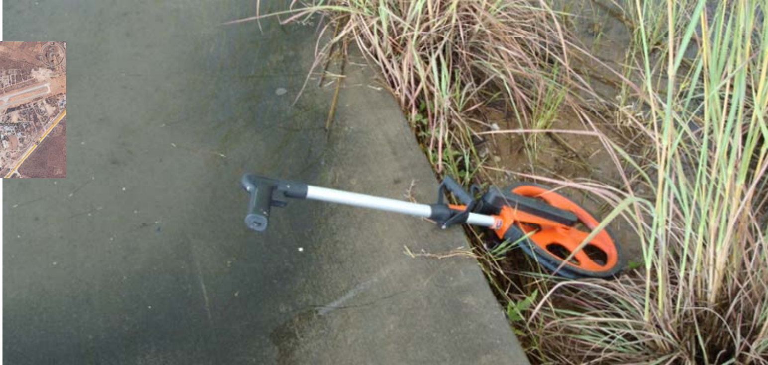
RA 8: Extent of step at 26 end due to erosion as well as vegetation
