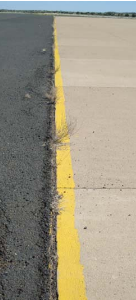
KA 12: Evidence of shoving of concrete slabs on passenger apron. Vegetation growth in cracks.
