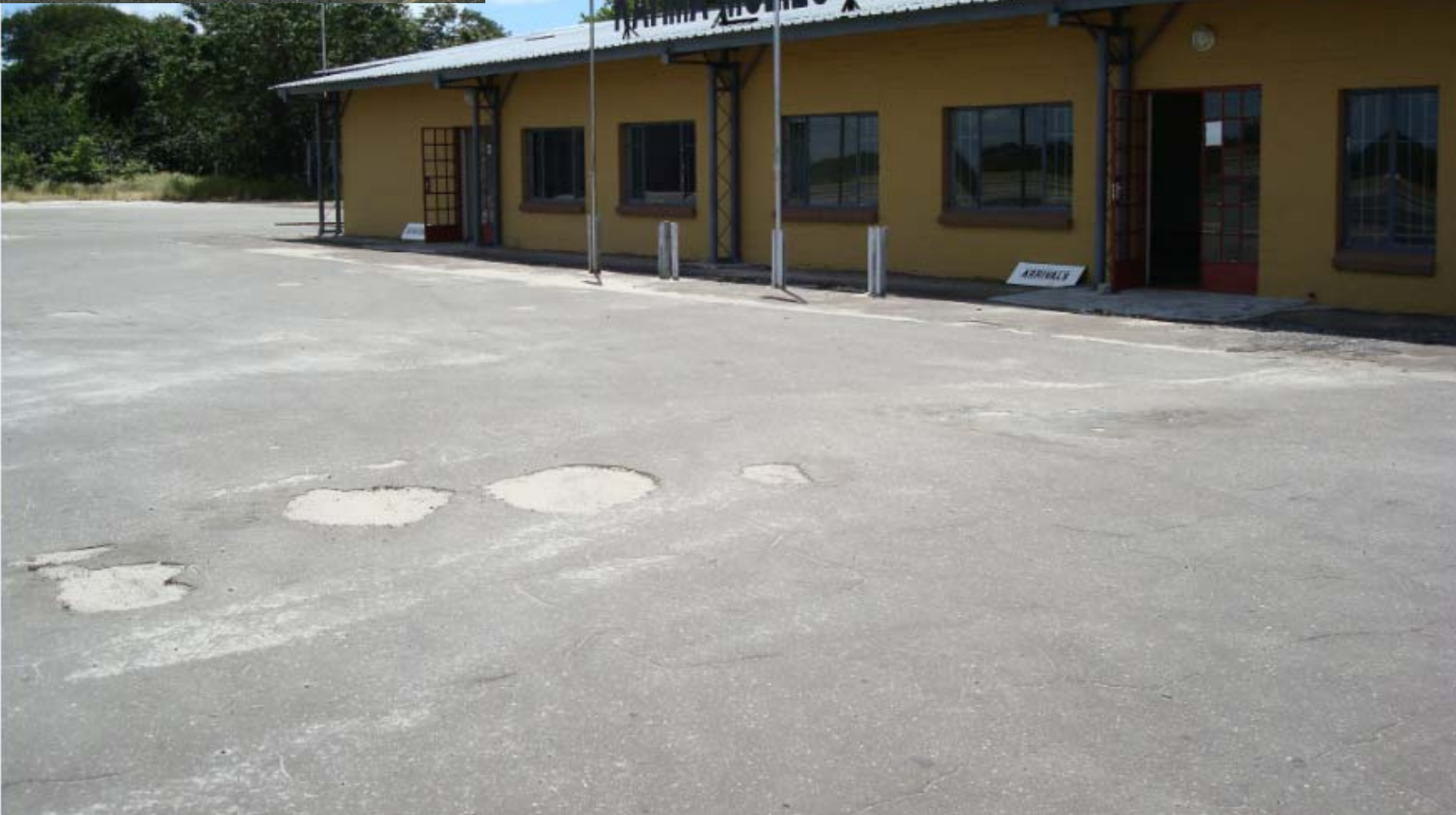
KMA : Potholes in front of passenger terminal
