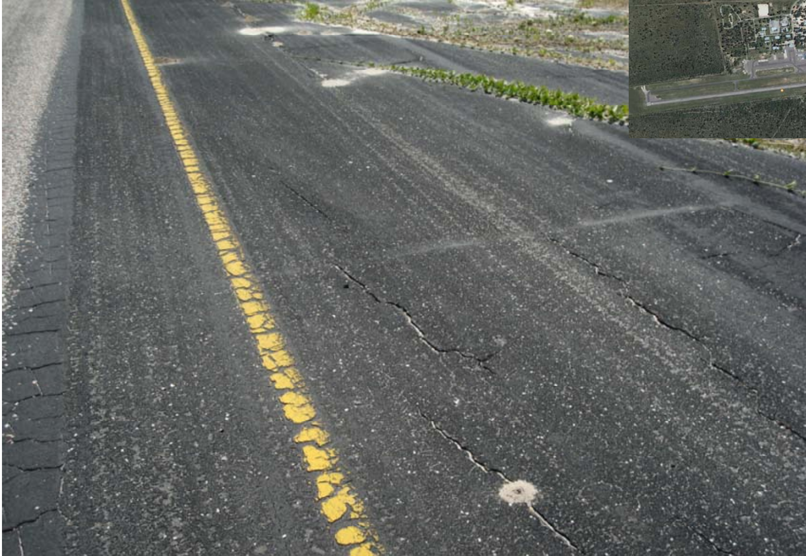
KMA 8: Shoulder at the 27 end showing ant activity, vegetation intrusion, longitudinal cracking on the shoulder and extreme map cracking on the paved area. Faint and fading line marking are also shown.
