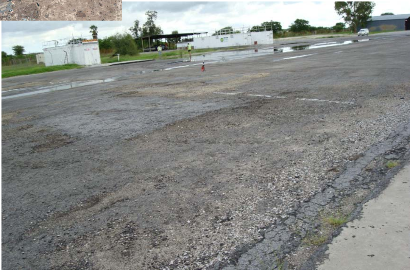
OA 2: Extent of ponding in front of modular refuelling units on area B. Extent of aging , ravelling and cracking in the foreground.
