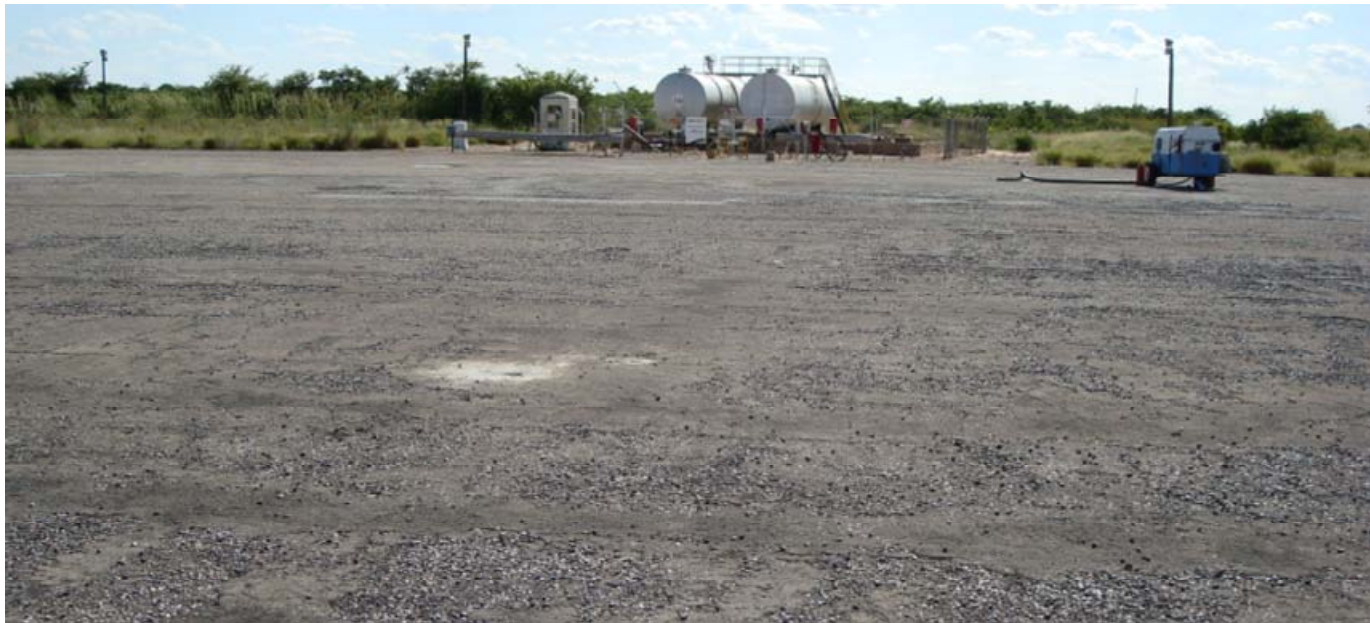
RA 4: Badly distressed area in front of refuelling area. Area has loose stones and potholes everywhere and is a FOD hazard. Mobile fuel pump in right hand side.
