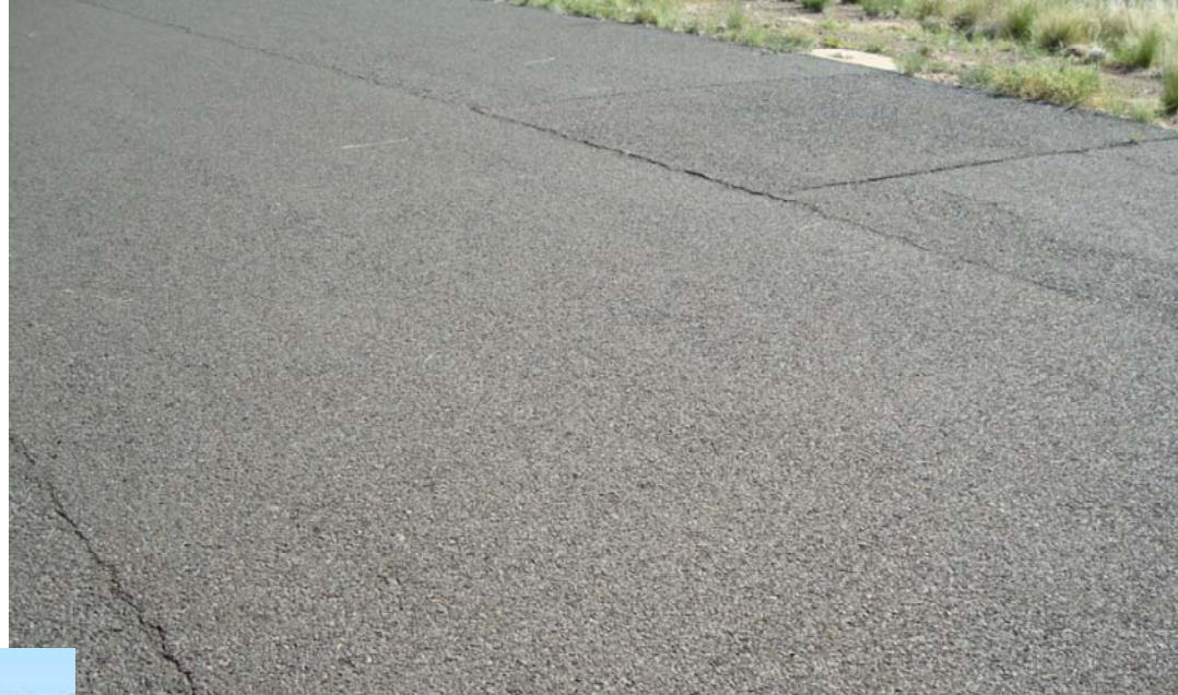
3: Longitudinal cracking and localised repair on shoulder.
