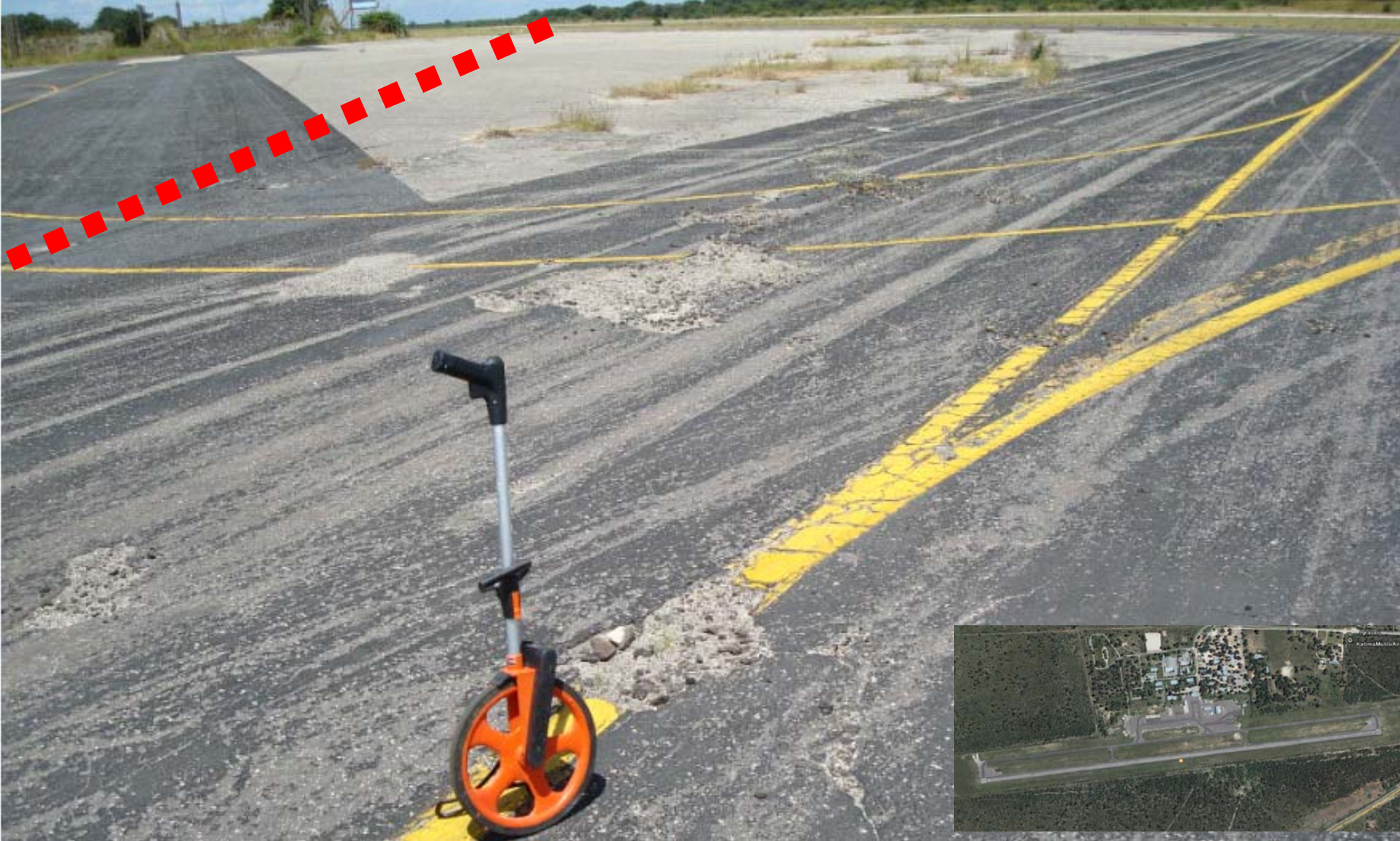
KMA 15: Current taxiway link with previous rejuvenation showing extensive potholing, cracking and aging. Suggested shorter taxi strive line (red dotted left) to cut out areas in need of rehabilitation as it will traverse over relatively sound areas.
