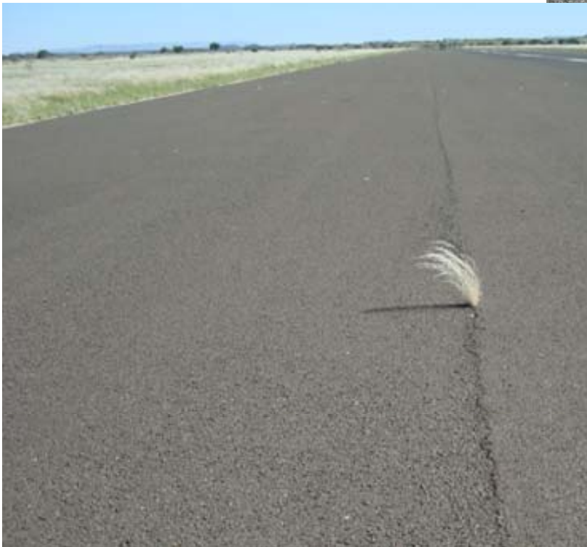
KA 6: Longitudinal cracking with vegetation in old construction joint on shoulder of main runway.
