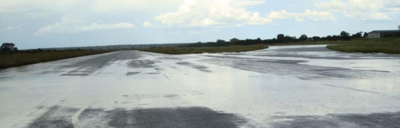
Figure RA 7: Sheet flow over main runway at RET and secondary runway intersection.
