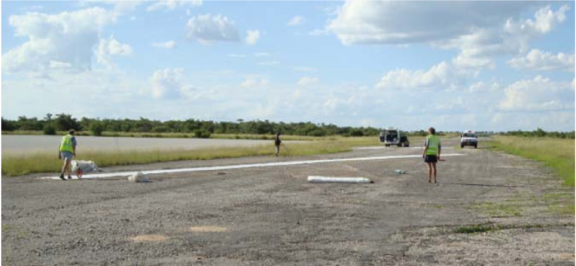
RA 6: Set-out of closure marking on secondary runway end. Discarded paved parking area is seen on the left hand side.
