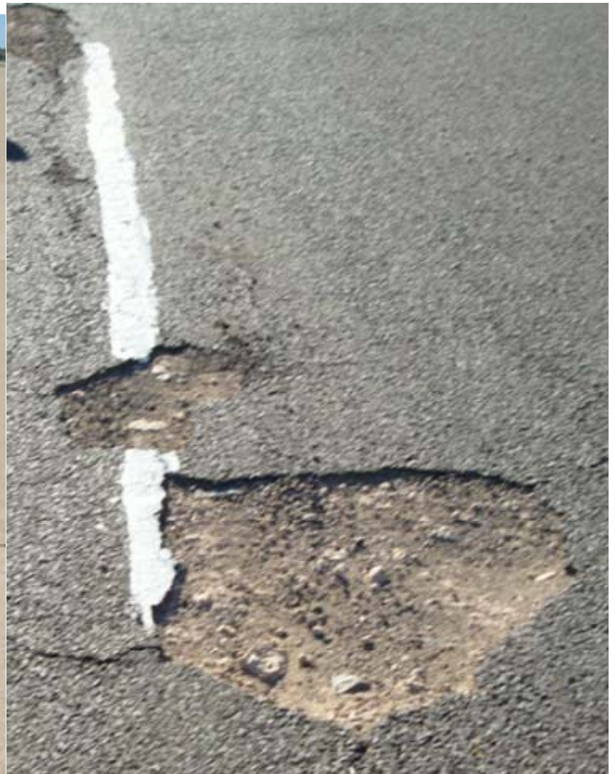
KA 11: Localised pothole on secondary taxiway.
