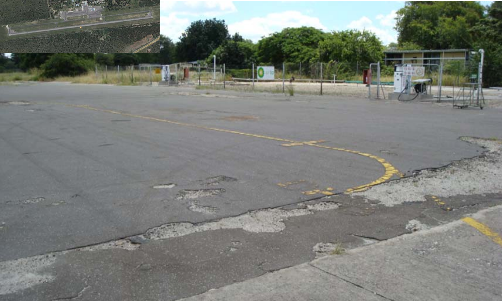
KMA 3: Cracked and potholed area at refuelling apron next to small concrete apron area in foreground.
