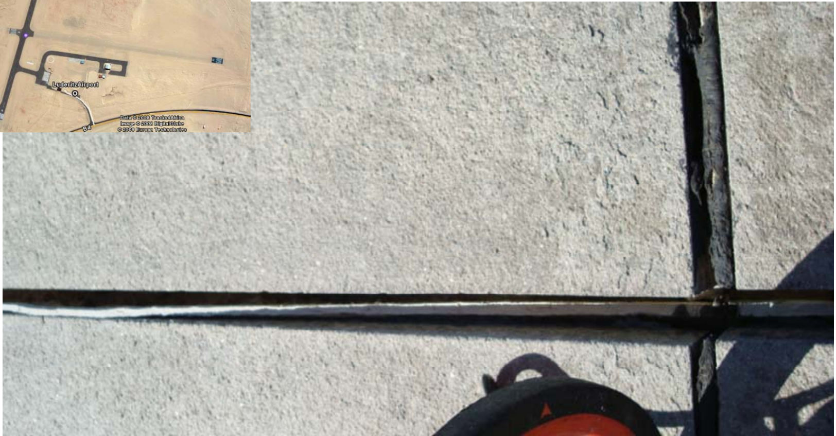
LA 7: Joint opening up due to movement of slab on passenger apron.
