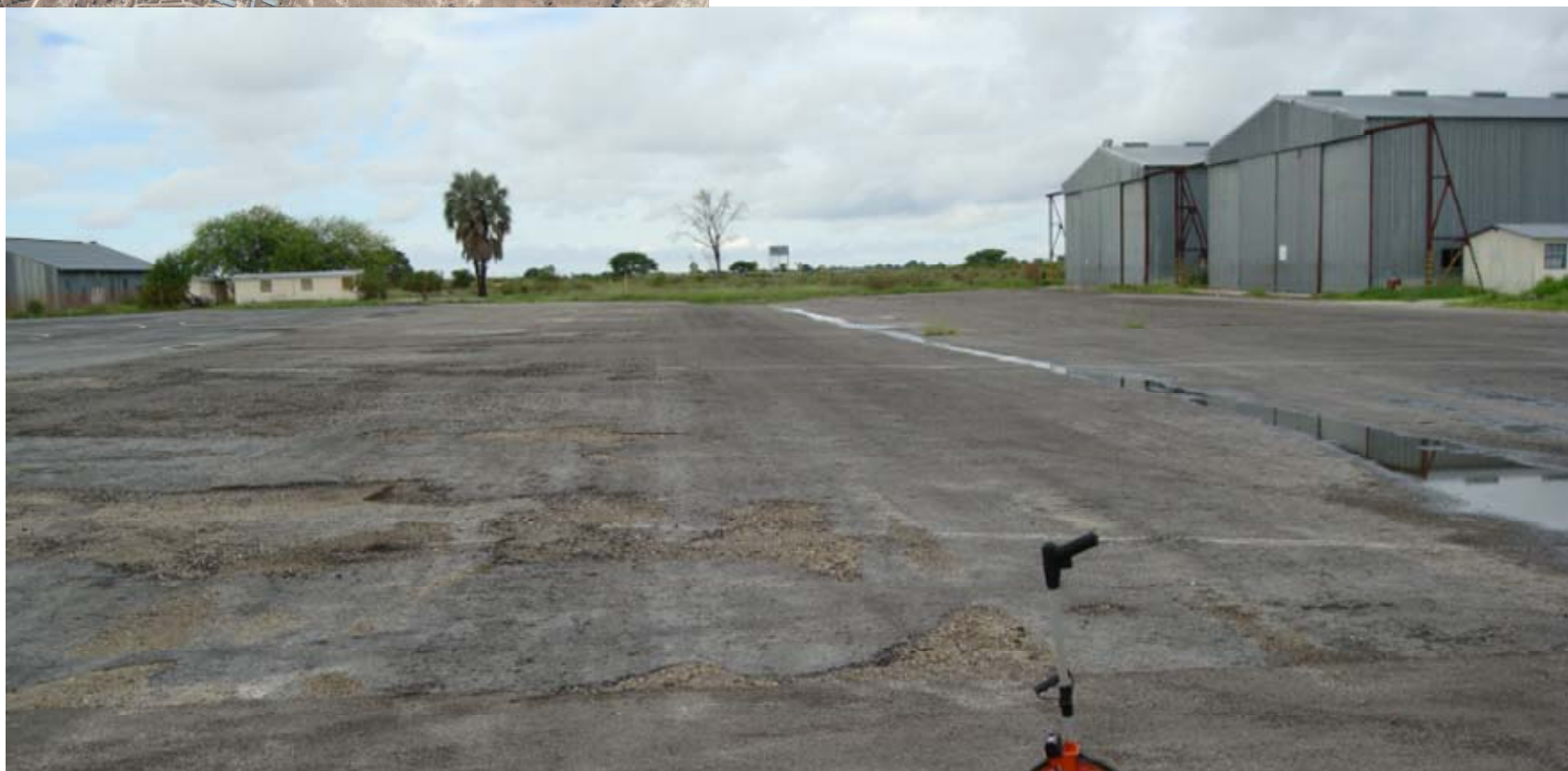
OA 22: Badly potholed and ravelling area A linking newly constructed refuel apron with area in front of large hangers. V type drain functioning in foreground.
