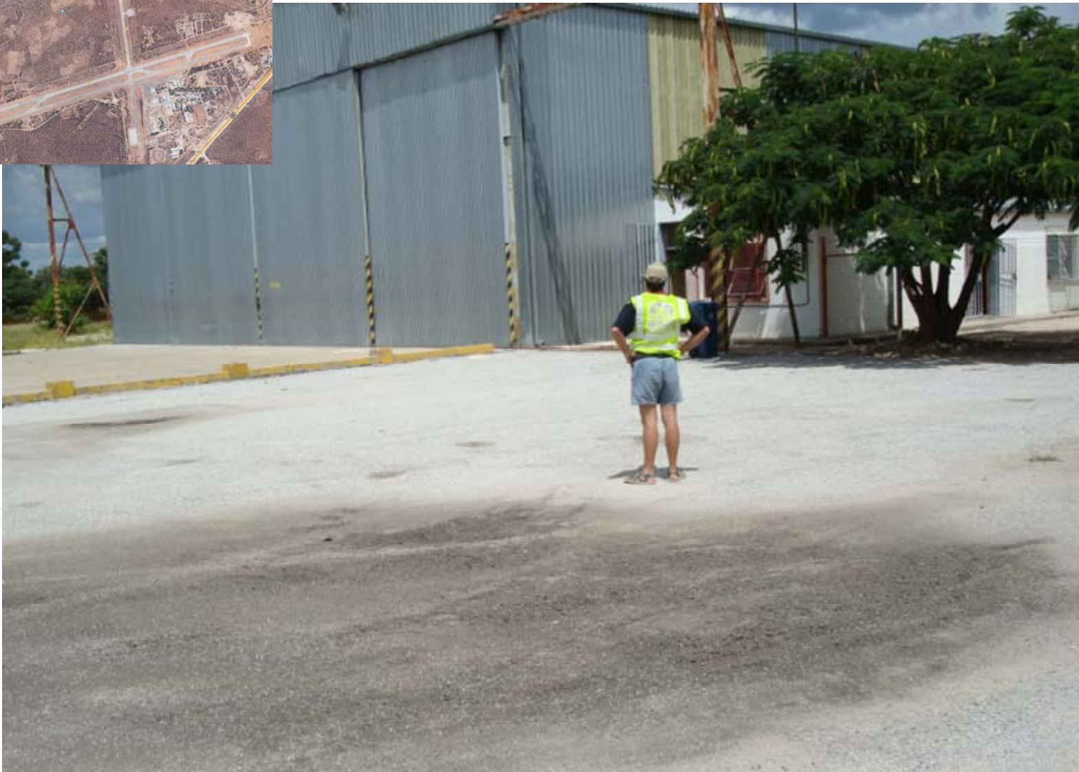
RA 1: Apron area in front of terminal building and hangar. Evidence of ponding seen in the foreground. Area under tree to the right was flooded during the subsequent rain storm.
