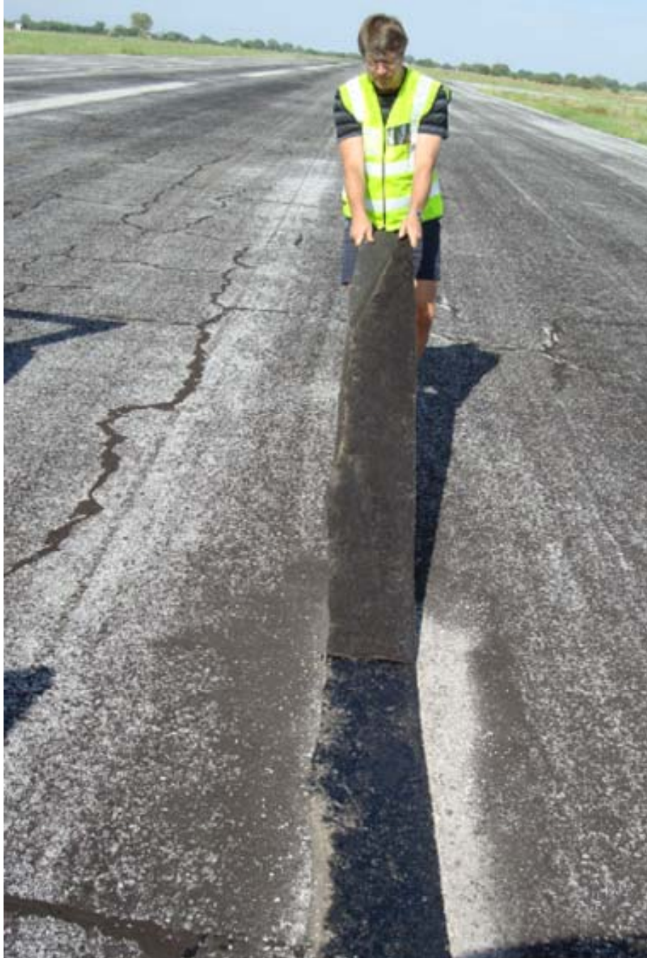
OA 14: Loose geo-fabric at 2007 crack sealing on shoulder. Extent of previous crack sealing and aged surface can also be seen.
