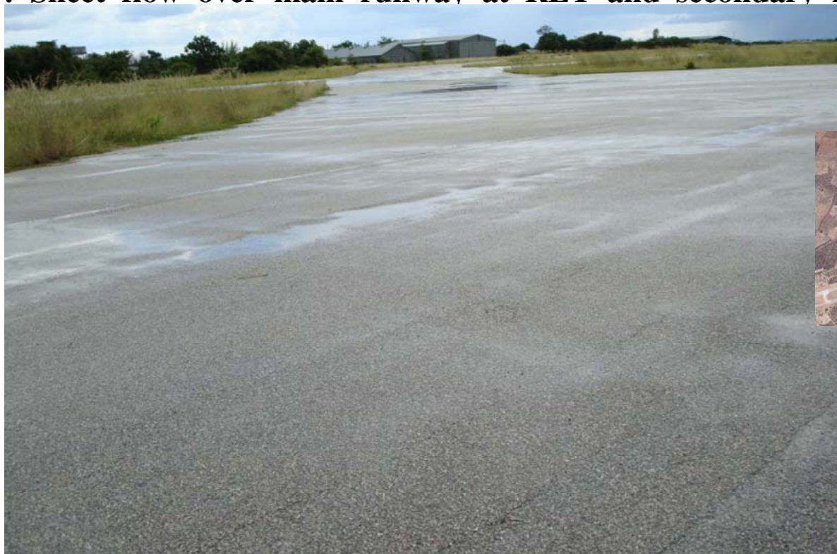
RA 10: RET on 26 end showing some ponding and longitudinal cracks in the foreground on the main runway
