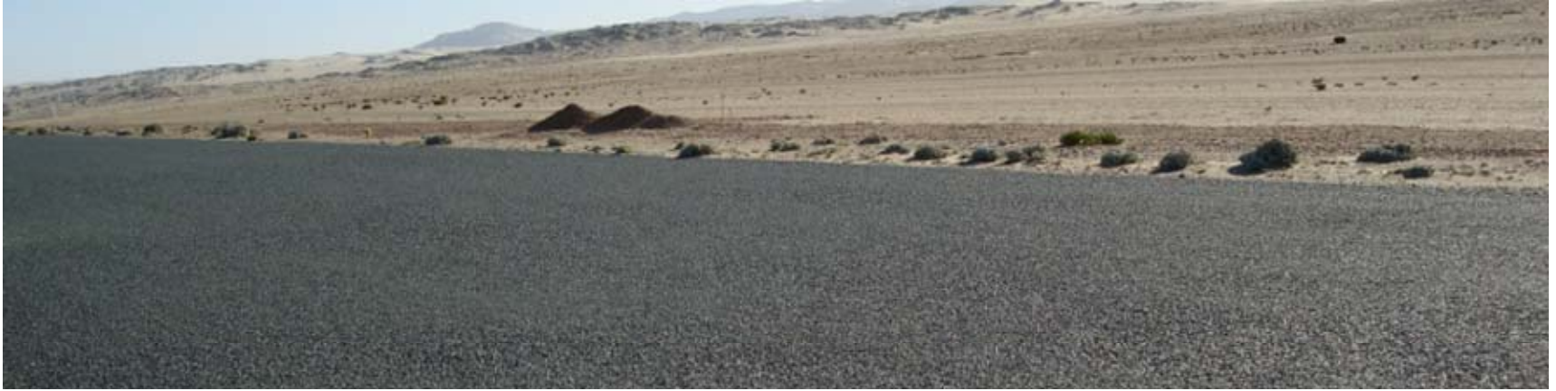
LA 13: Small bush and shrubs on runway edge causing minor sand deposits due to “wind shadow”. These shrubs are to be removed.
