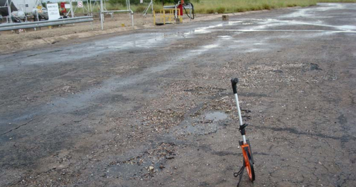
RA 12: Potholes and loose gravel extent plus extreme cracking on refuelling apron area directly after rain storm.
