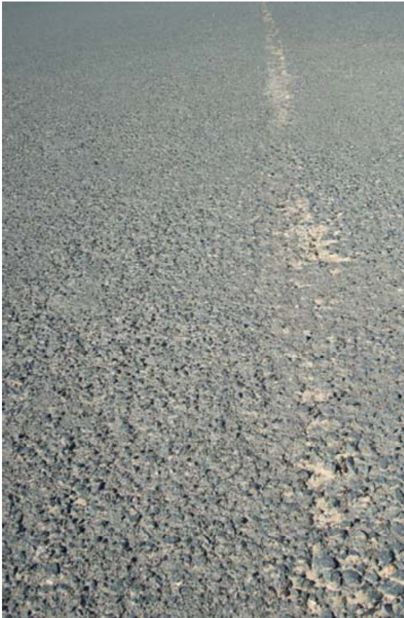
LA 5: Localised construction joint at main runway 04 end in need of repair via crack filling.
