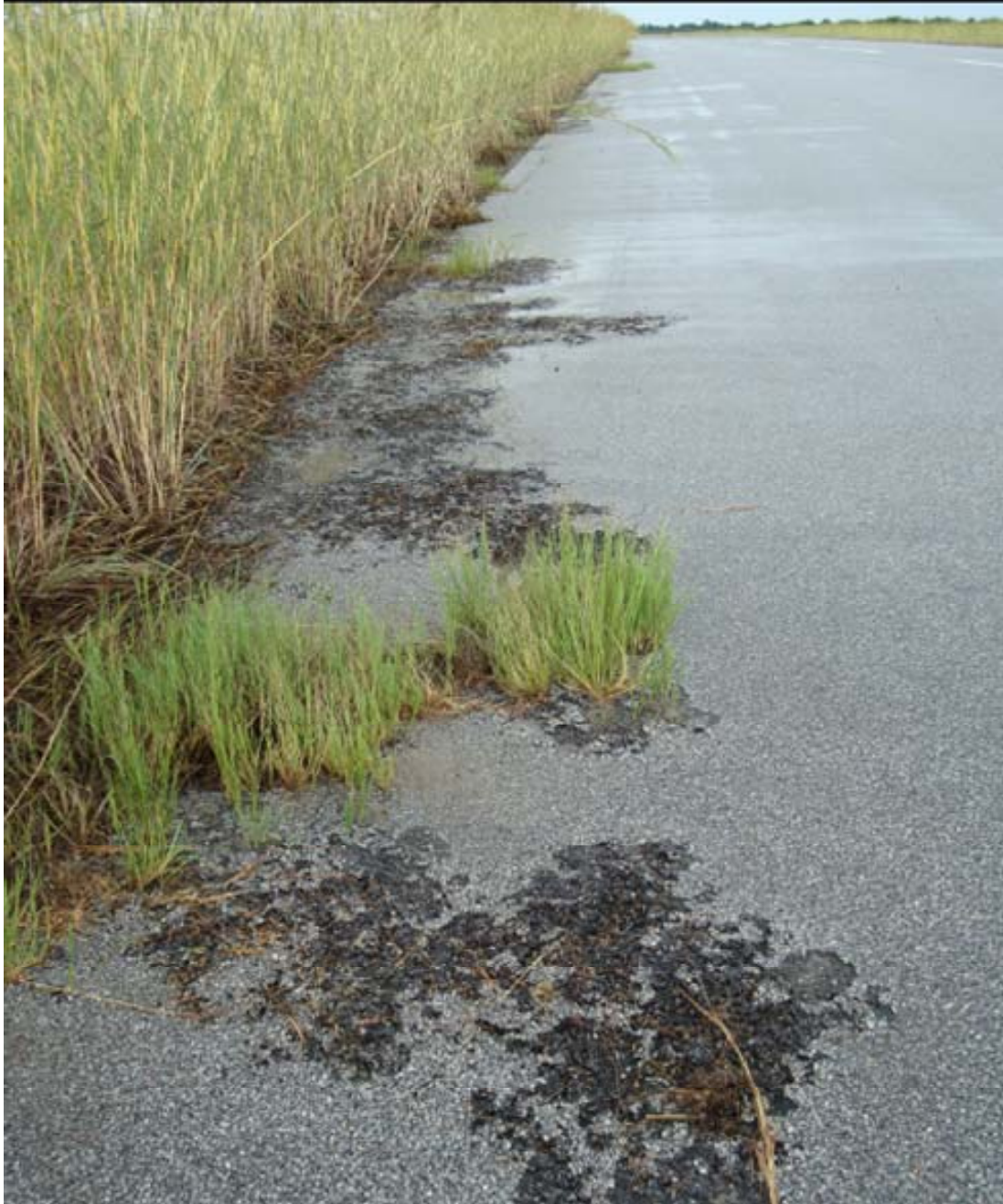
RA 3: Intrusion and break up of shoulder asphalt area due to vegetation and high grass on shoulder blocking side drainage.
